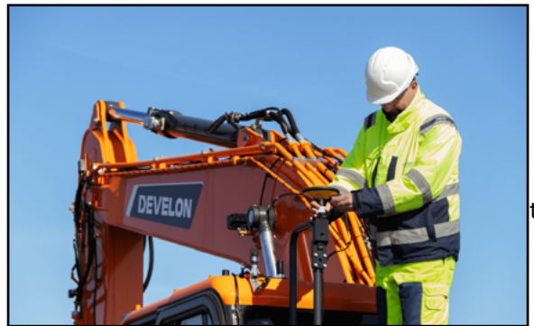
Let's start by installing a machine guidance system on this excavator. Leica
